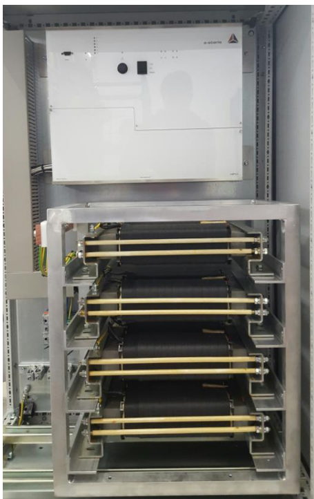
Figure 151: Current injection in control cabinet for indoor installation
